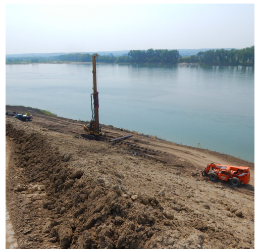
Above left: Rock key / trench being installed (Photo by Dwayne Walker); Above right: Pipe piles being installed (Photo courtesy SHSND)
