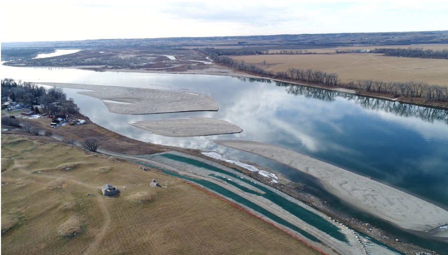
Overview of the south end illustrating the reshaped bank where the rotational slumping occurred (Photo by Dwayne Walker)
