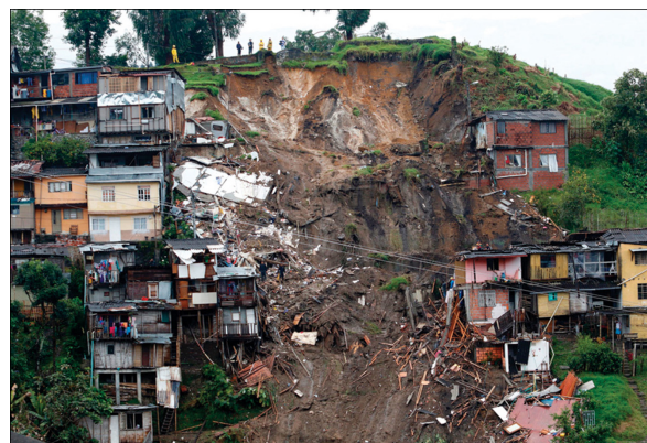
Landslide in Colombian rural community (Daniels 2017).
