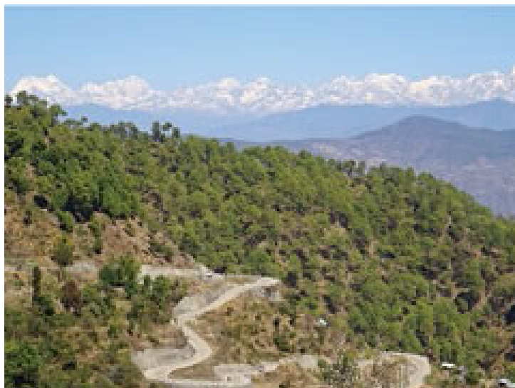
The Sindhuli Road meanders through the Mahabharat Range, with the Himalayas in the background. (Photo: Nippon Koei Co., Ltd.)
