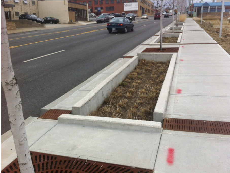
Photo 1. Curb Cuts into landscaped bioretention cell – Photo courtesy of USACE, Kansas City District
