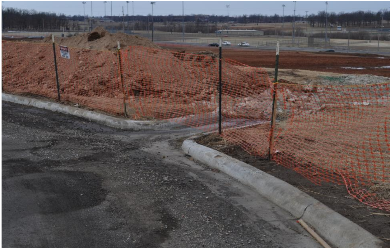
Photo 6. Road debris will end up in storm system (Corner of 5 th and Michigan) – Photo courtesy of USACE, Kansas City District
