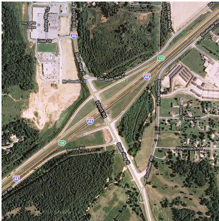
Image 2. Possible West Gate Park and Ride Location at Exit 156 on Interstate 44 – Image courtesy of Google Earth (© 2011 Google)
