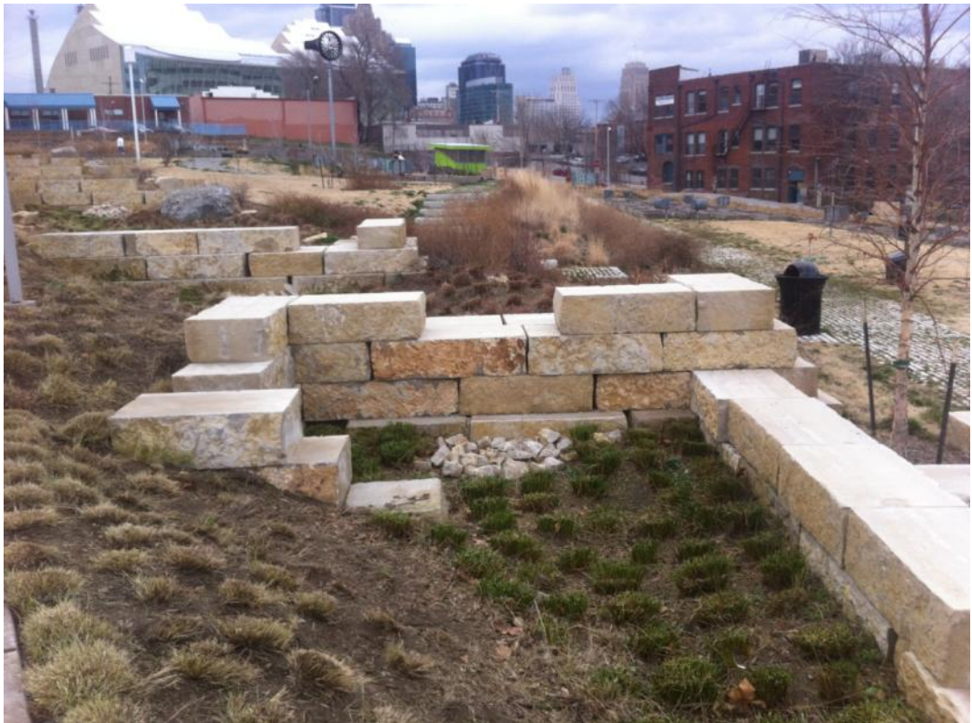
Photo 10. Bioswale / Bioretention Areas with Checkdams – Photo courtesy of USACE, Kansas City District
