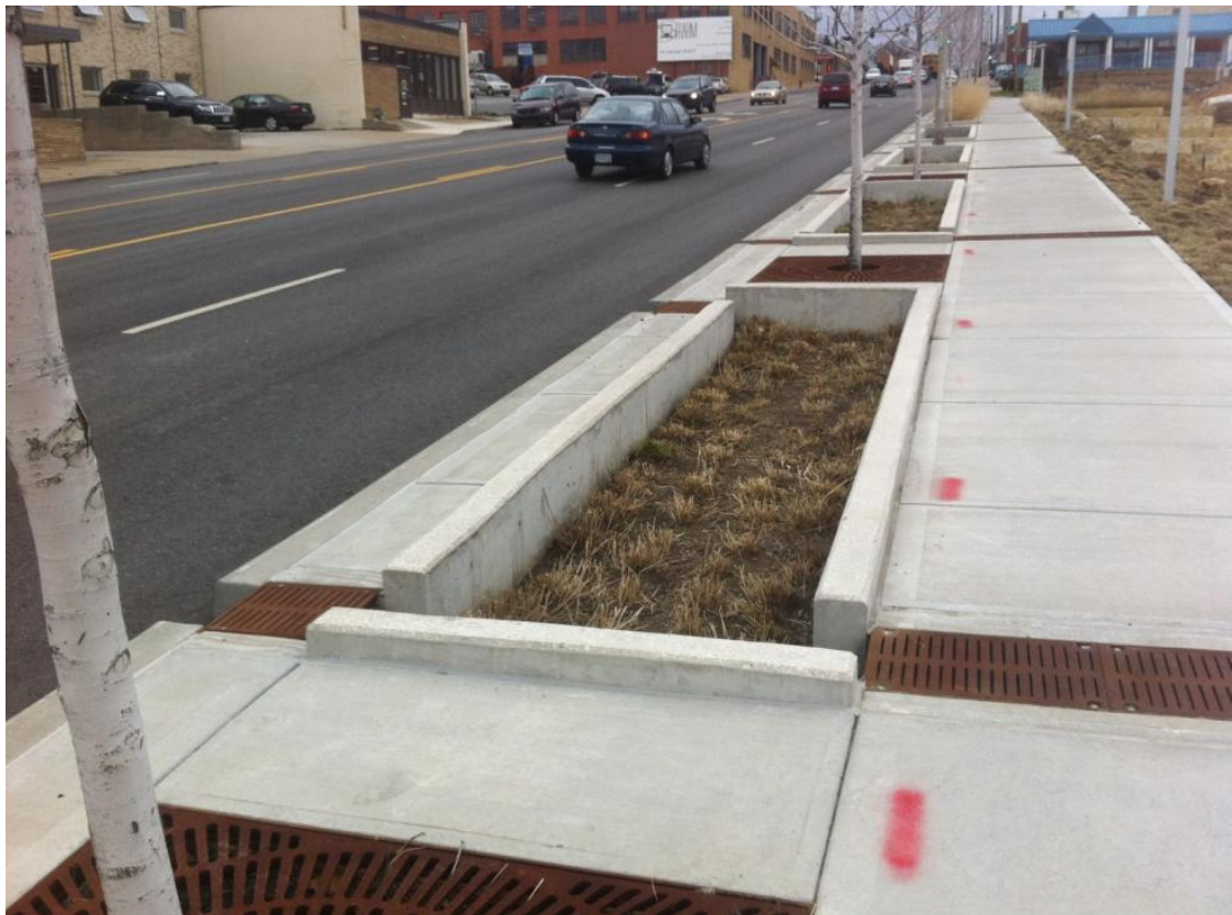
Photo 11. Green Street Example. Pedestrian friendly and bioretention characteristics – Photo courtesy of USACE, Kansas City District
