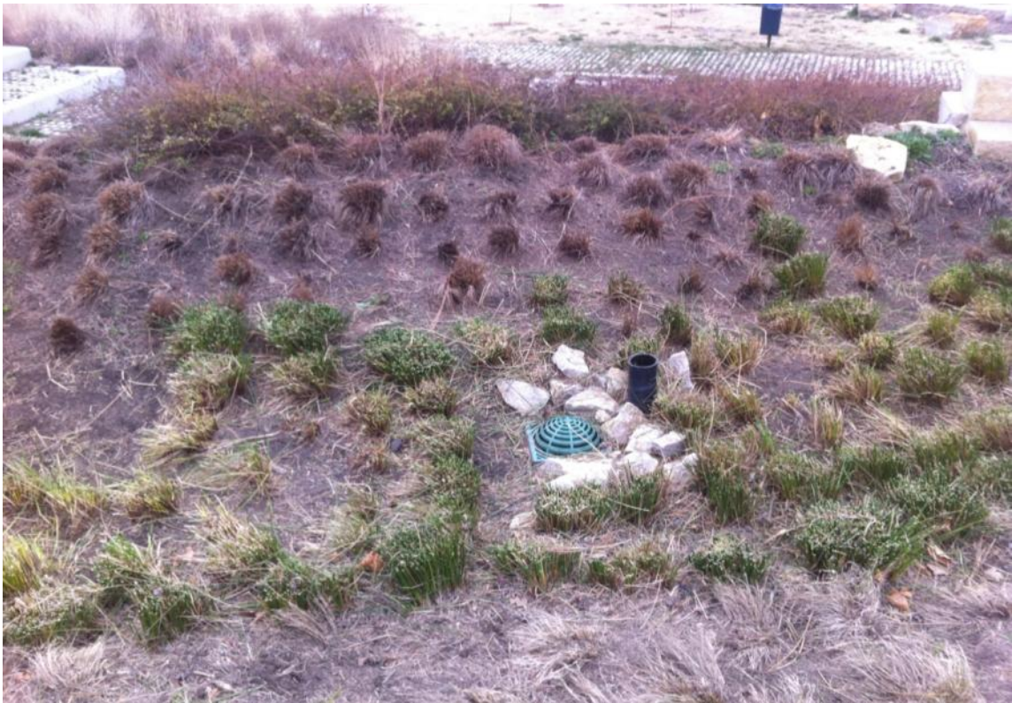
Photo 9. Bioretention System with Grasses – Photo courtesy of USACE, Kansas City District
