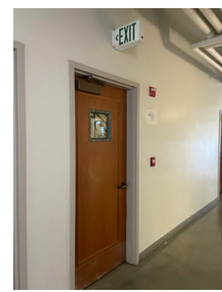
IMAGE 2: STREISINGER EXIT STAIR
