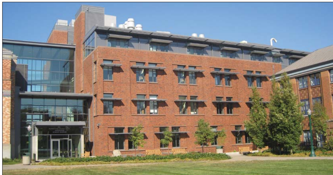
Exterior of the recently opened Robert and Beverly Lewis Integrative Science Building.
