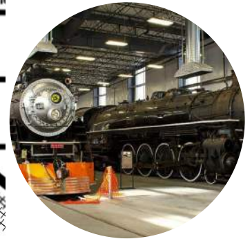
It is a new engine-house that house historic locomotives as well as a visitor center and an interpretive center.
