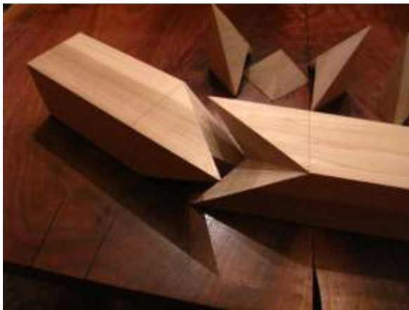
Bird's Mouth Joint from BrokenRiverJoinery.wordpress.com
