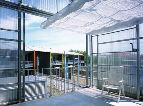
porch, polycarbonate balcony
