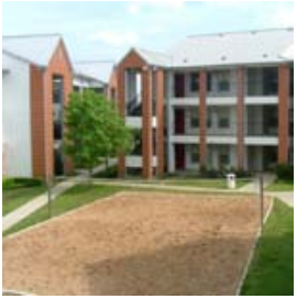
Figure 2-4 A view of the courtyard at the Century Court Apartments. Image at centurycourt.com .
